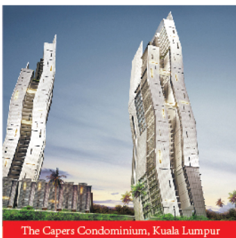
The Capers Condominium, Kuala Lumpur
